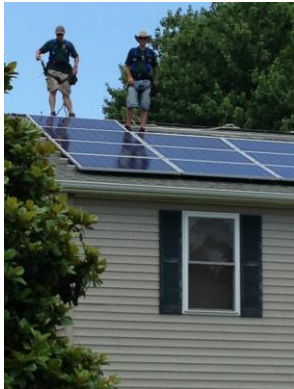
Two of our certified professionals installing a 5kw roof system
